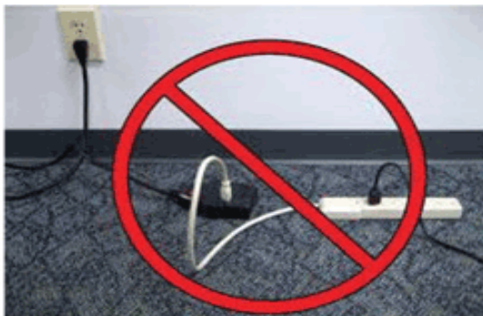
Daisy-chained multi-plug outlets
